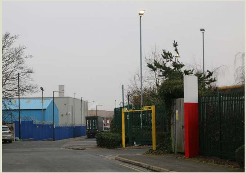
Collett Way, Great Western Industrial Estate
