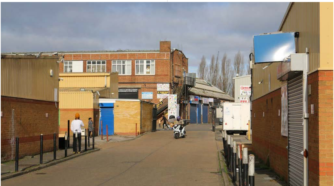
Southall Enterprise Centre, Bridge Road
